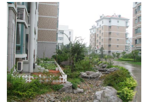
In the foreground is an efficient - and attractive - kerb-side drainage system, instead of a simple gutter. Photo: Bob Cook
