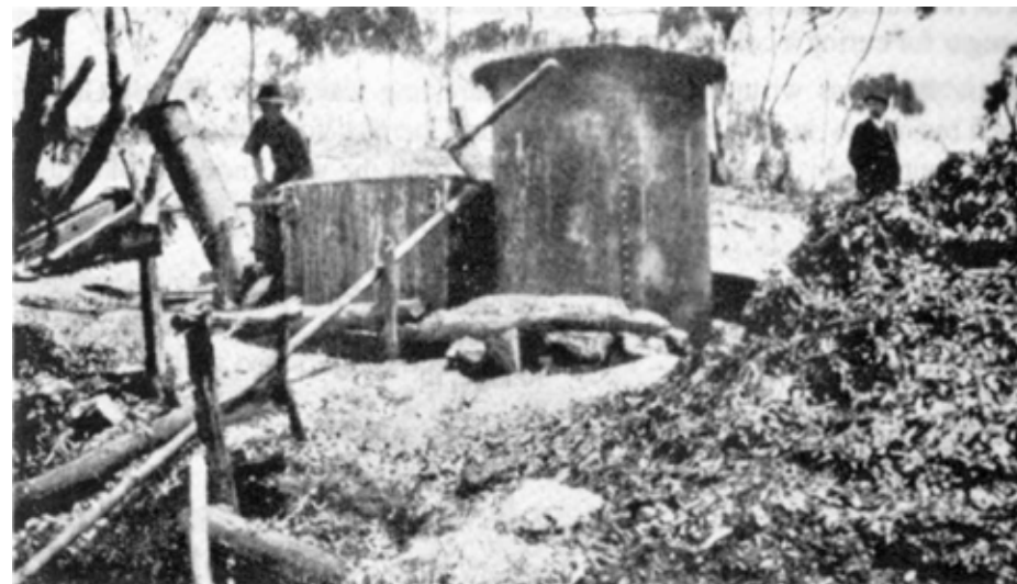
Fig. 1. Crude still for distillation of eucalyptus oil
